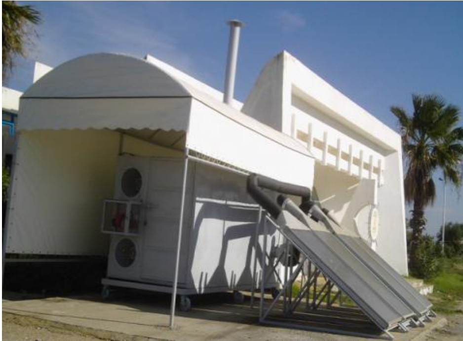
Fig. 1. Overall view of the solar-gas tunnel dryer pilot.
